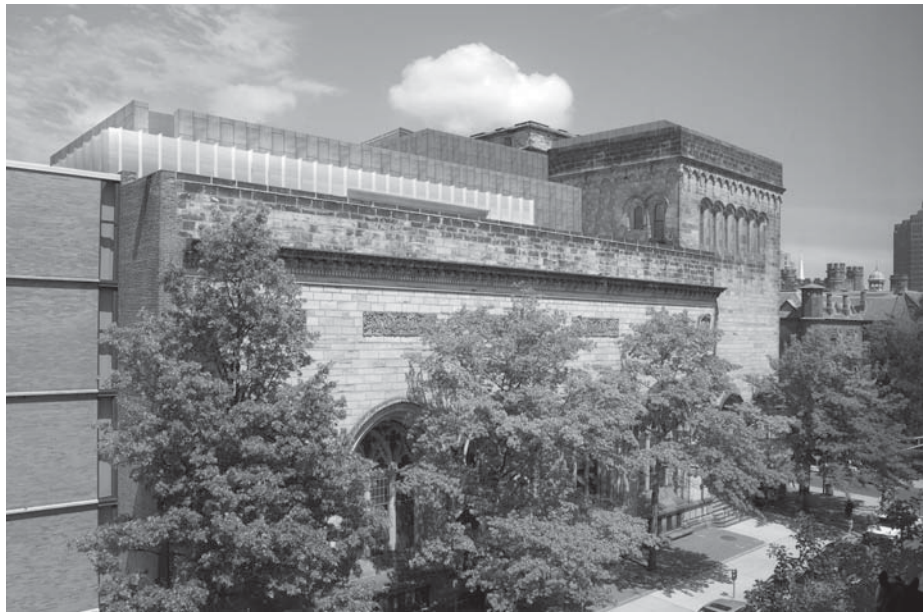
Yale University Art Gallery, Louis Kahn building, view of west window-wall. (c) Elizabeth Felicella, 2006
